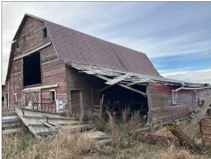
Photo 4.10-1. Feature 1, Site 32MO1740 red barn, facing southwest.
