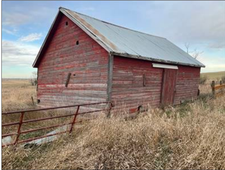
Photo 4.10-2. Feature 2, Site 32MO1740 historic shed, facing northwest.
